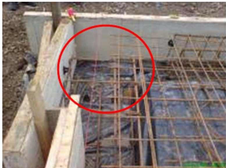
Missing reinforcement
