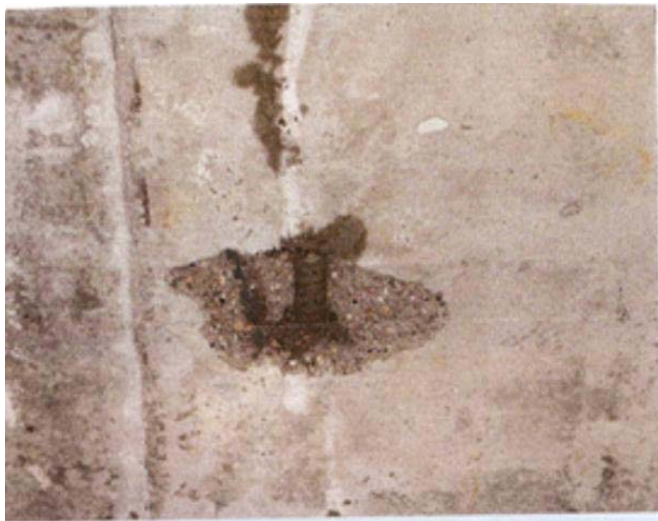
Soffit of slab showing pre-stressing duct
