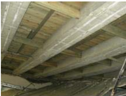
Concrete beams above
