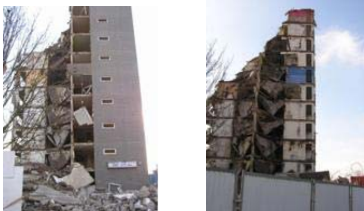
Photographs of the collapse of the third LPS block
