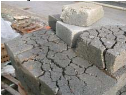
Cracked concrete blocks
