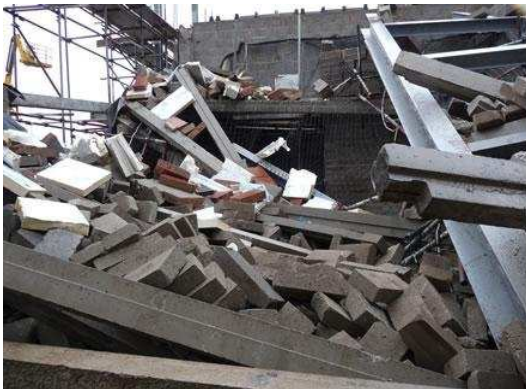
Part of the collapsed office block
