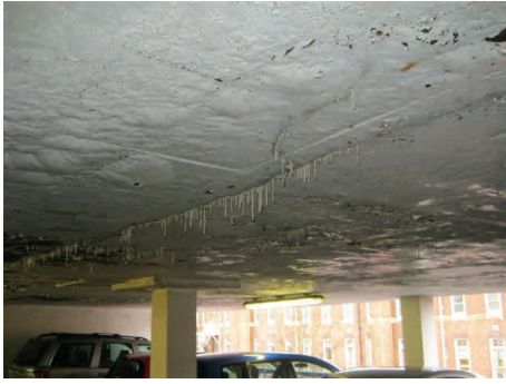
Soffit deterioration
