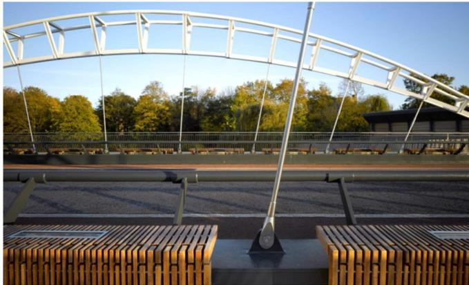
*Figure 1* Typical tension rod with end connector used on a bridge (**not** from a CROSS report)
