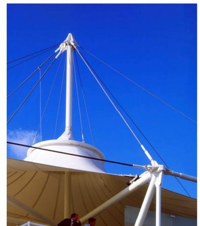
*Figure 2* Typical tension rod with end connector used on a building. (**not** from a CROSS report)
