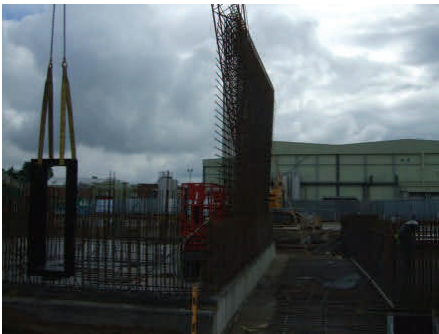
A rebar cage similar to those referred to above
