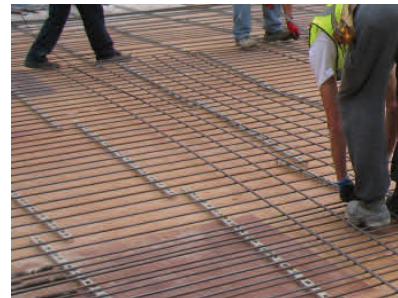
Example of bad practice – spacers laid in continuous lines
