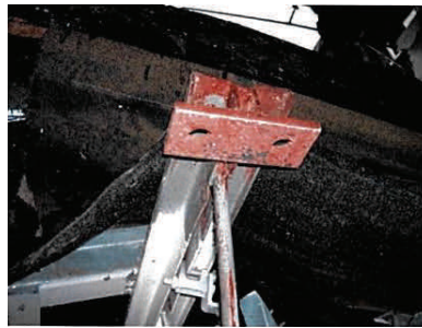
End fixing of truss to cleat
