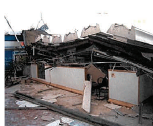
Collapsed roof
