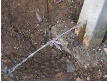
Water released from a stanchion (reproduced with permission)
