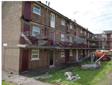
Fall of 2 nd floor balcony onto 1 st floor (reproduced with permission)
