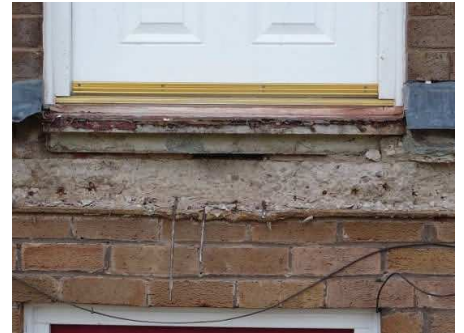
Rebar in the bottom of cantilever slab (reproduced with permission)
