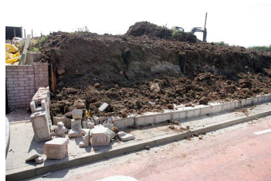
Wall with soil on one side
