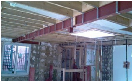
Three Span Beam with Columns Removed
