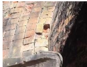
553 Spalling masonry
