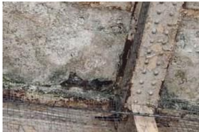
549 Spalling concrete
