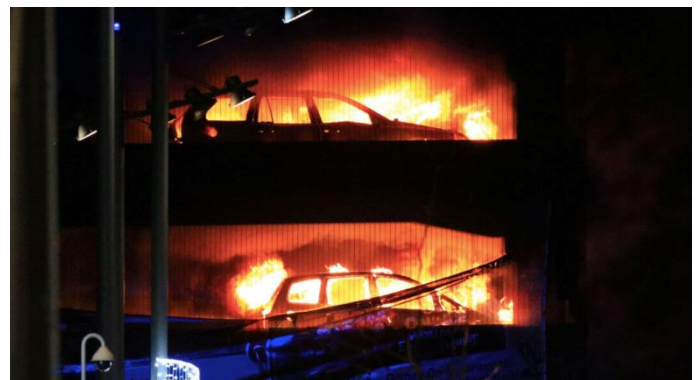
Figure 2: Fire on separate levels. Image courtesy of Liverpool Fire and Rescue Services (MFRS).
