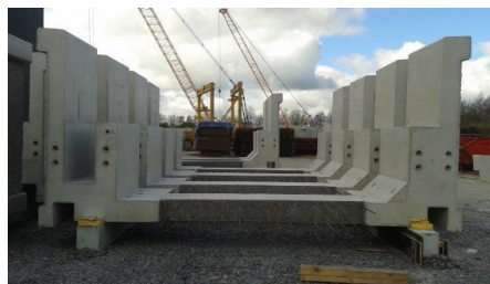
● Figure 2 U-shaped precast kerbs
