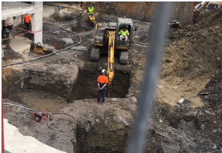
Figure 1 Excavation hazards
