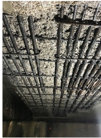
● Figure 3 Hydro-demolition
