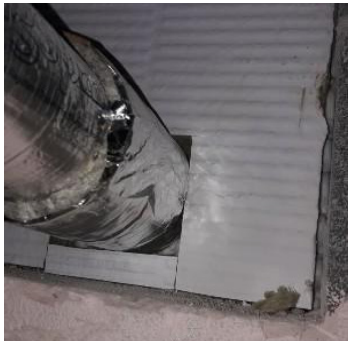
Figure 1: single thickness batts cut to fit around services and into openings
