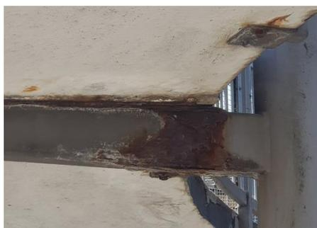
Figure 1: corroded cantilever deck support
