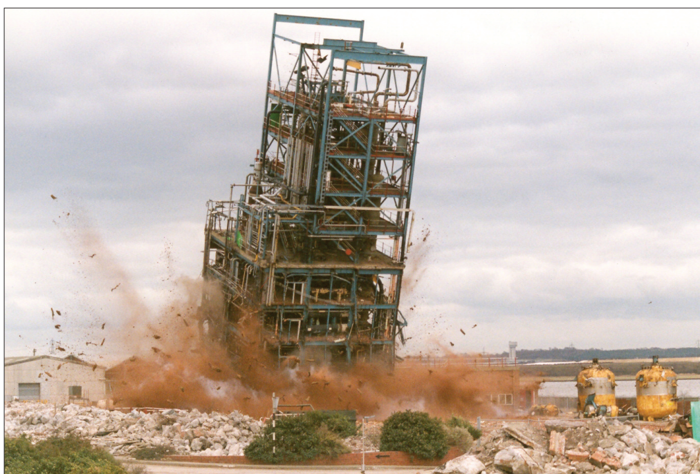
The explosive demolition of the Paraquat distillation column at Widnes.
