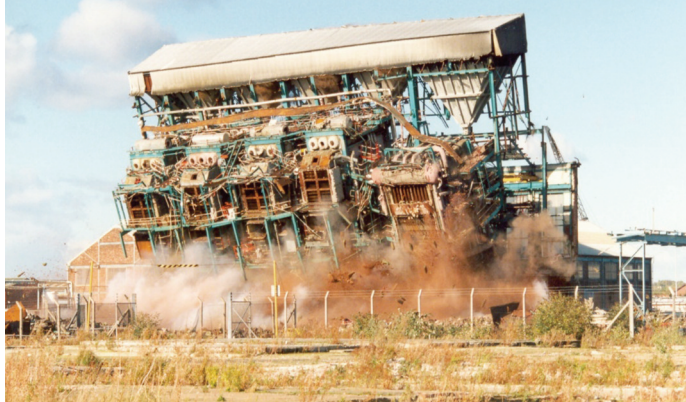
Demolition of the five coal-fired boilers on former chemical manufacturing site at Widnes. Copyright J Wolstenholme ©
