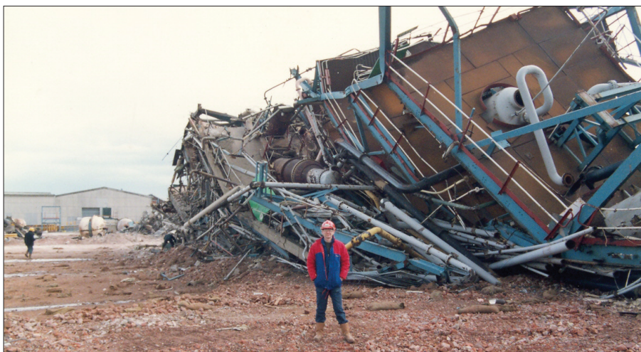
The author in front of the demolished Paraquat Tower.
