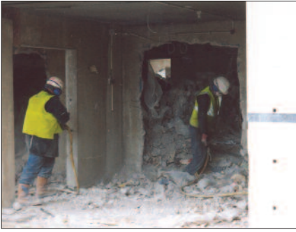
Wall drilling to RC walls.
