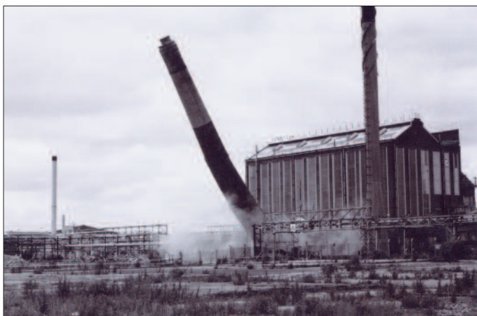
Masonry chimney on chemical works.
