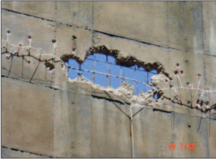
Test blast on thin shelled wall of cooling tower.
