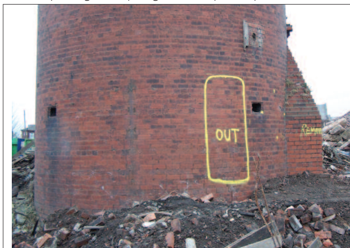
Preliminary setting out of openings on masonry chimney.
